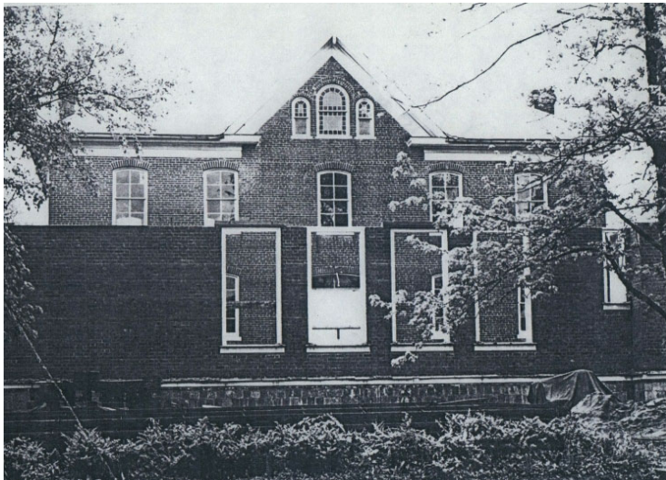
LOOKING FROM BROAD STREET IS A PHOTO OF THE NEW ST. JAMES SCHOOL CONSTRUCTION GOING UP WITH THE OLD SCHOOL IN THE BACKGROUND. THE ORIGINAL 1905 SCHOOL WAS COMPLETELY TORN DOWN IN 1947.
